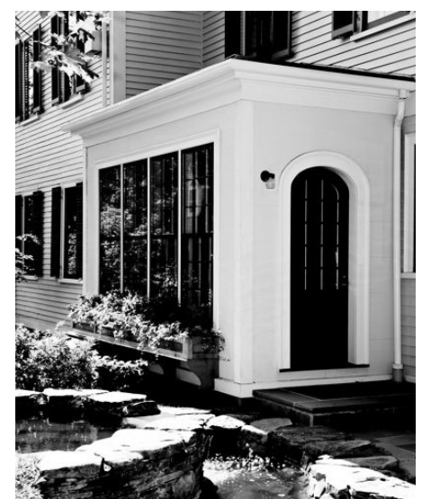
When restoring a historic home like this one in Cambridge, Mass., it is essential to maintain the home's integrity and accuracy.
